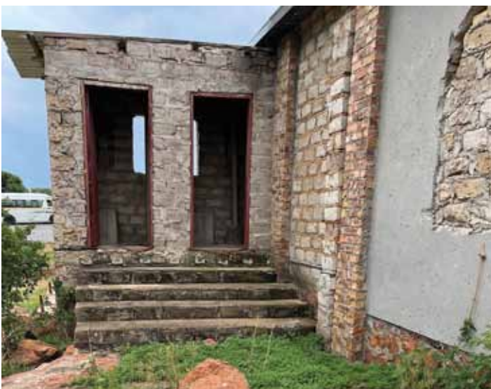
Two restrooms attached to the sanctuary.
